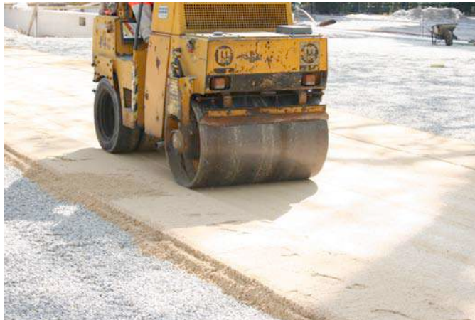
Do not allow material to dry completely before rolling
